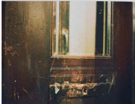
Lift (with selftape), Helmsdorferstrasse
